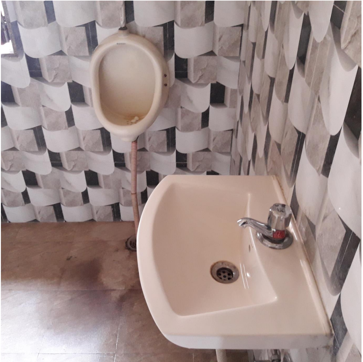
Staff Room Wash Room
