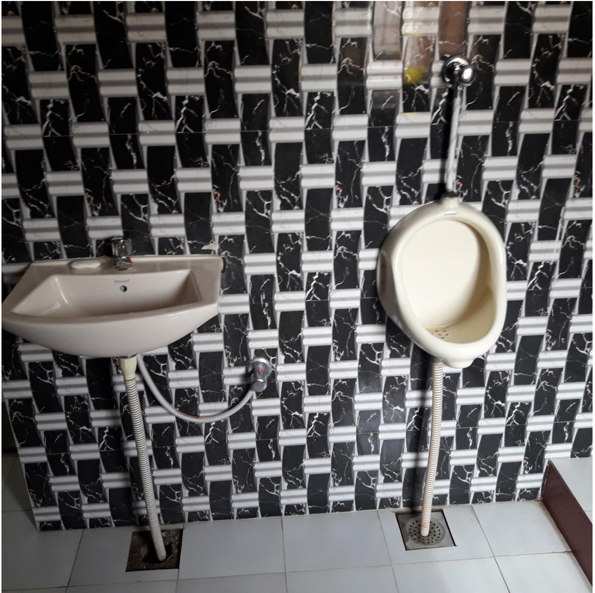
Office Wash Room
