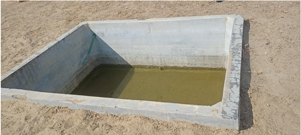
Tank for collection of Surface run-off water
