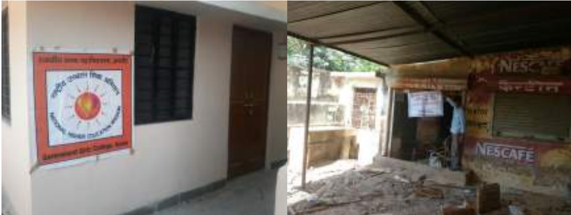
New construction LABORATORY before & after
