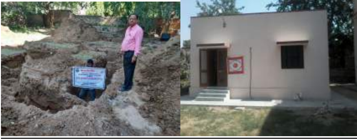
New construction hostel warden residence before & after
