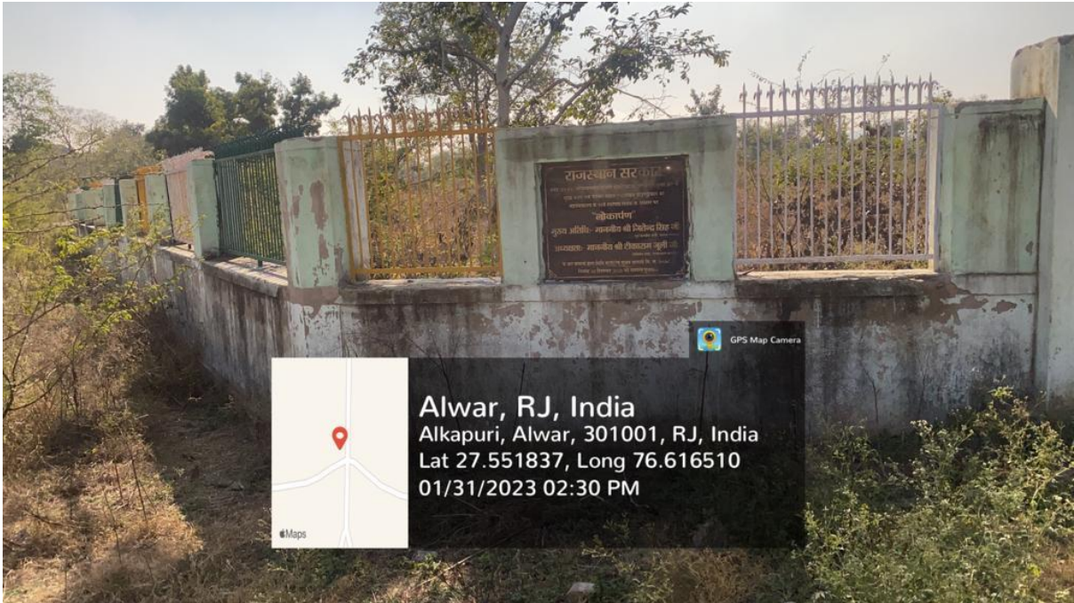
Cement Wall Fencing
