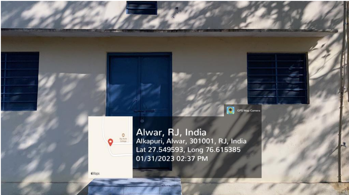
Renovation of Chemistry Lab
