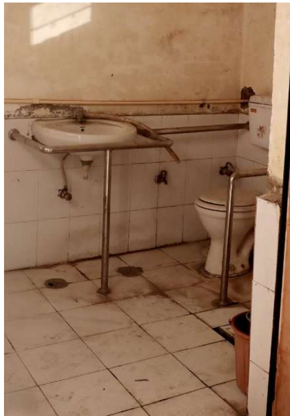
Disabled friendly Washrooms
