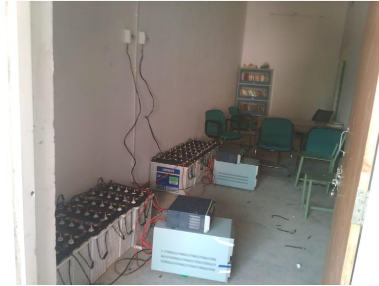
7.1.2 SOLAR BATTERY UNIT
