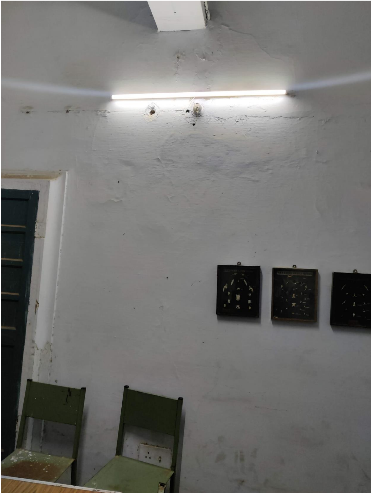
7.1.2 LED LIGHTS IN CLASSROOMS AND LABS
