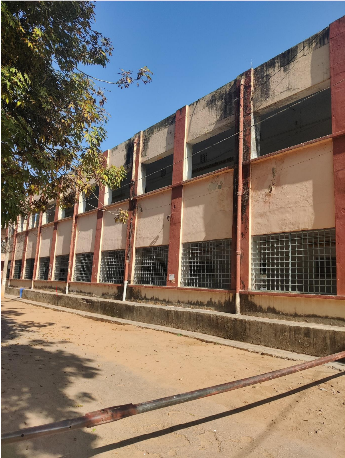
7.1.4 Rain water harvesting (Drains from Roof connected via Pipelines to underground storage tank )
