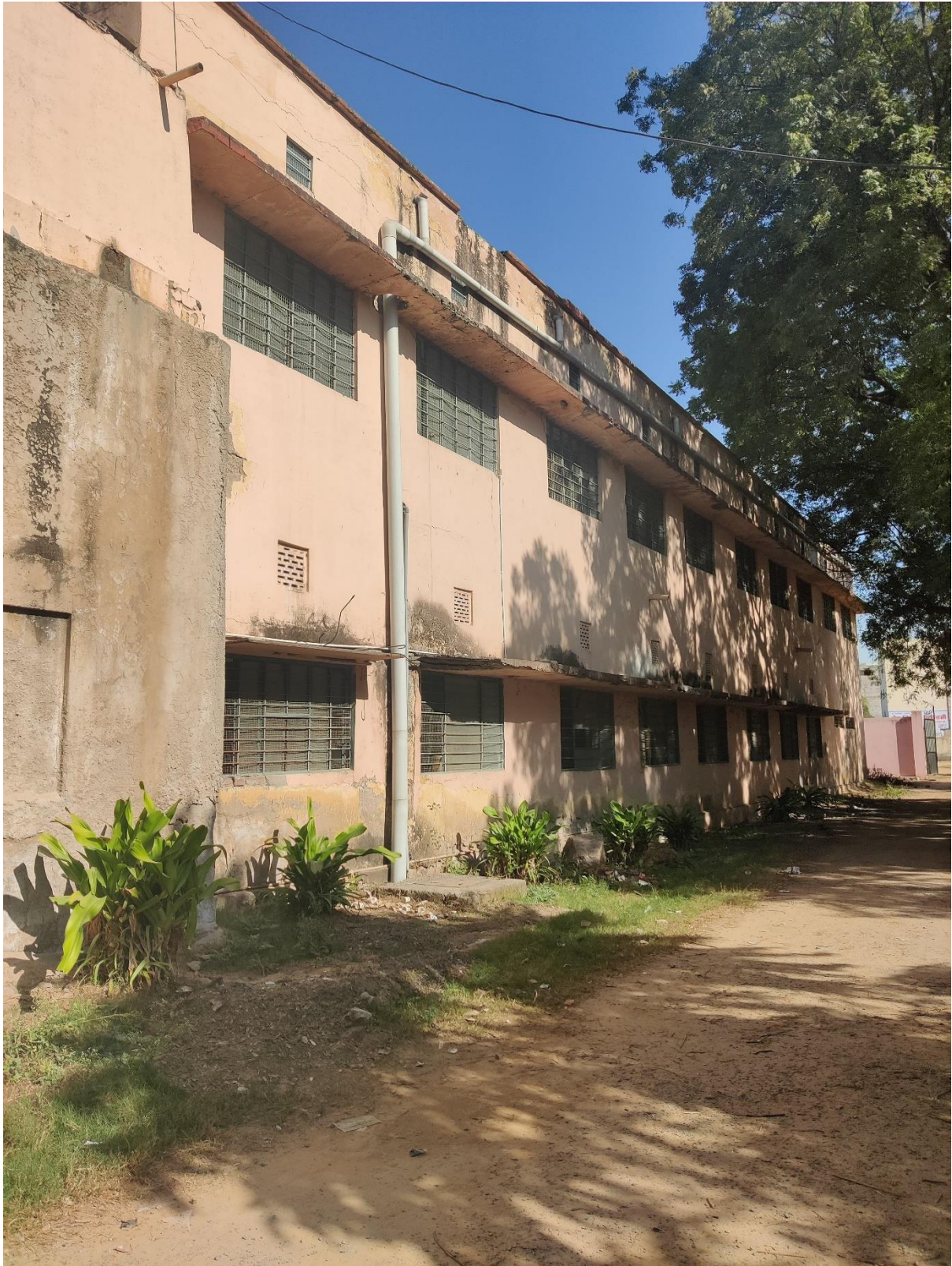
7.1.4 Rain water harvesting (Drains from Roof connected via Pipelines to underground storage tank )
